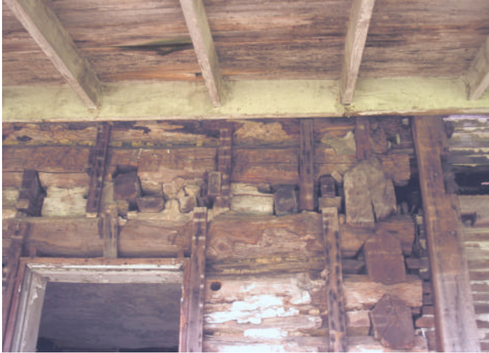
Figure 20. Detail of joists projecting through the façade of the Isaac and Margaret Sharp house. The only original joist in this photograph is the square joist almost centered over the window. The other joists were filled in later.
