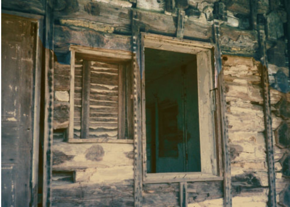
Figure 16. Front door opening at Isaac and Margaret Sharp house. Original small window opening with later door and larger window openings to left and right. The original window was covered over when the new larger window was added.
