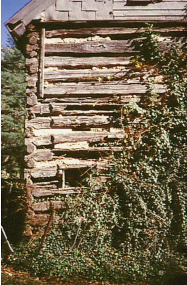
Figure 18. Detail from visible gable-end of the Isaac and Margaret Sharp house. Small window opening that would have provided light in a first-floor pantry.
