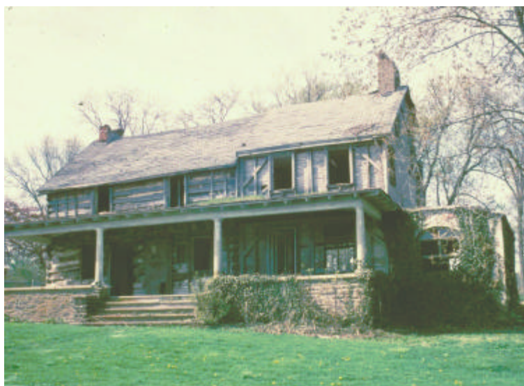
Figure 22. Isaac and Margaret Sharp house with frame addition built during the ownership of Isaac Sharp, son of the first Isaac Sharp. Concrete and stone room (to the right) is a still later addition.
