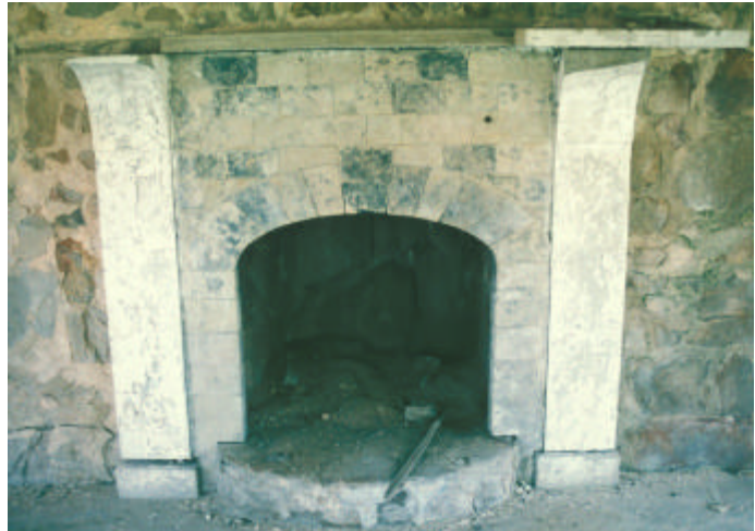
Figure 31. Fireplace in the concrete and stone “sun room”—a very late addition to the Isaac and Margaret Sharp house.
