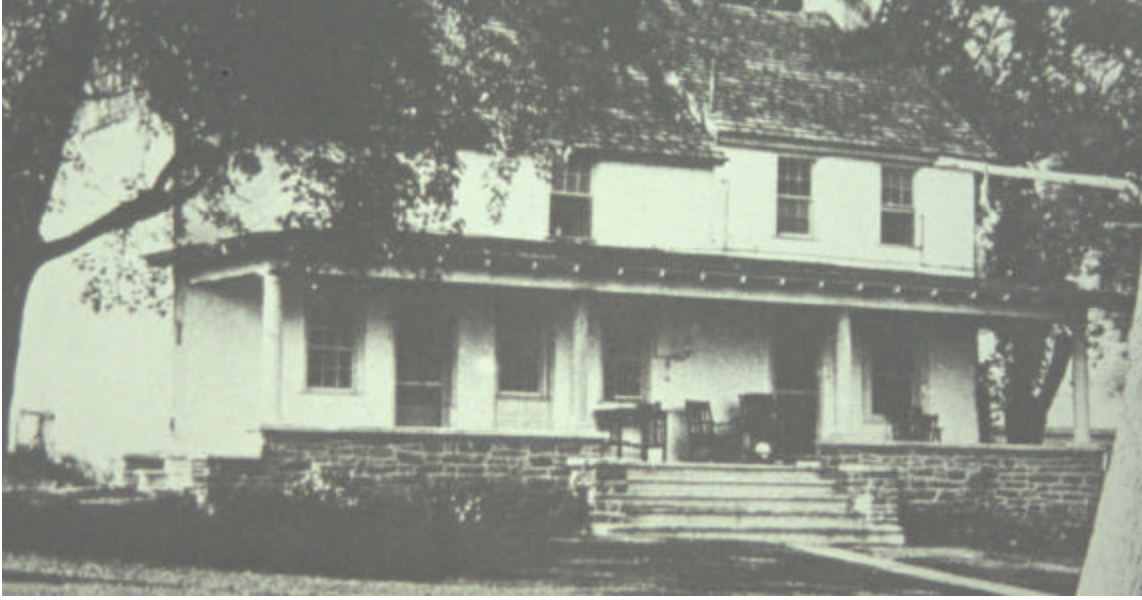
Figure 27. Photograph of the Isaac and Margaret Sharp house with its nineteenth century addition. A coat of stucco united the log and frame facades. Photo may date to the early twentieth century. Photo from Eakins in Avondale, p. 17.
