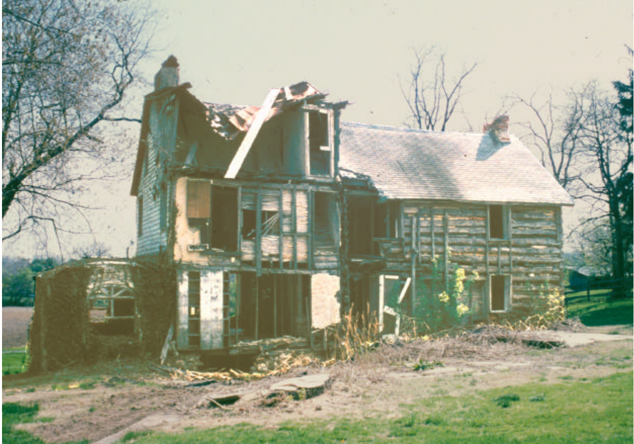
Figure 9. Rear view of Isaac and Margaret Sharp house with subsequent additions.
