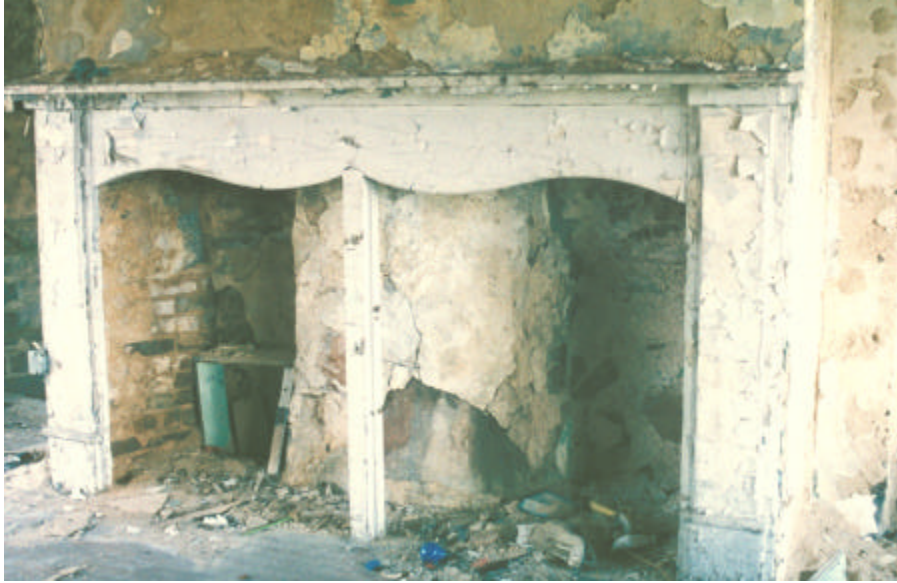
Figure 33. Fireplace in the first-floor front room of the nineteenth-century frame addition to the Isaac and Margaret Sharp house. The masonry that projects into the back of the fireplace is part of the adjoining fireplace in the “sun room.”
