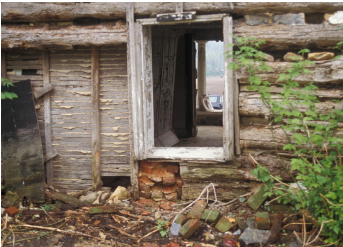
Figure 17. Detail from rear of the Isaac and Margaret Sharp house. Originally, this area consisted of a door-window combination. The window was located to the right and is still evidenced by a vertical piece of window framing. The door was located to the left and is evidenced by the brick in-fill and a notched area in the lowest surviving log. Both the door and window were later replaced by a single larger window.
