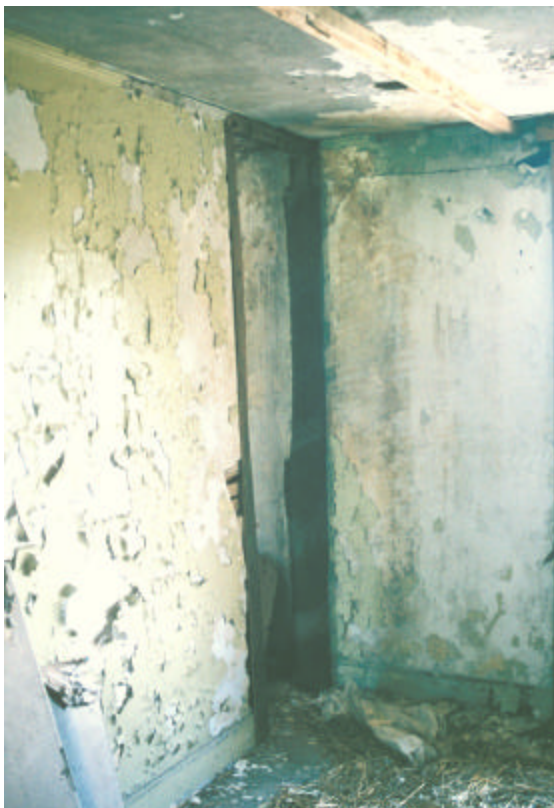
Figure 32. Plaster walls and ceiling on the second floor of the original log portion of the Isaac and Margaret Sharp house. The plaster on the walls and ceiling was laid over lath, which was applied to the logs and joists that first formed the visible walls and ceiling.
